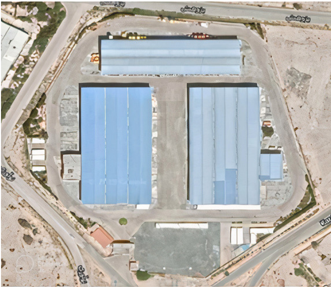
Fig. 2. Industrial campus in Kish Island
