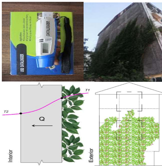
Fig. 1. Measured Green wall in the east direction.
