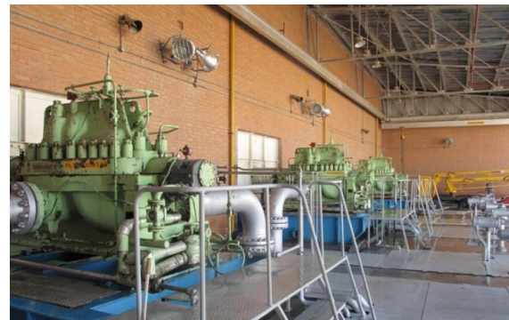
Fig. 2. View of the pumping station.
